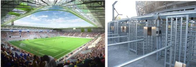
In case the answer for both questions is yes, the BioSec system receives the member ID and the person puts its hand onto the BioSec terminal (at the gate) to read out its biometric ID. In case there is a matching with the previously recorded, we grant access to the stadium.
